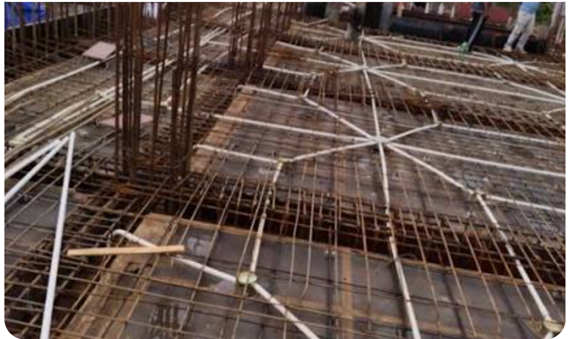
Electrical Work (Slab)
