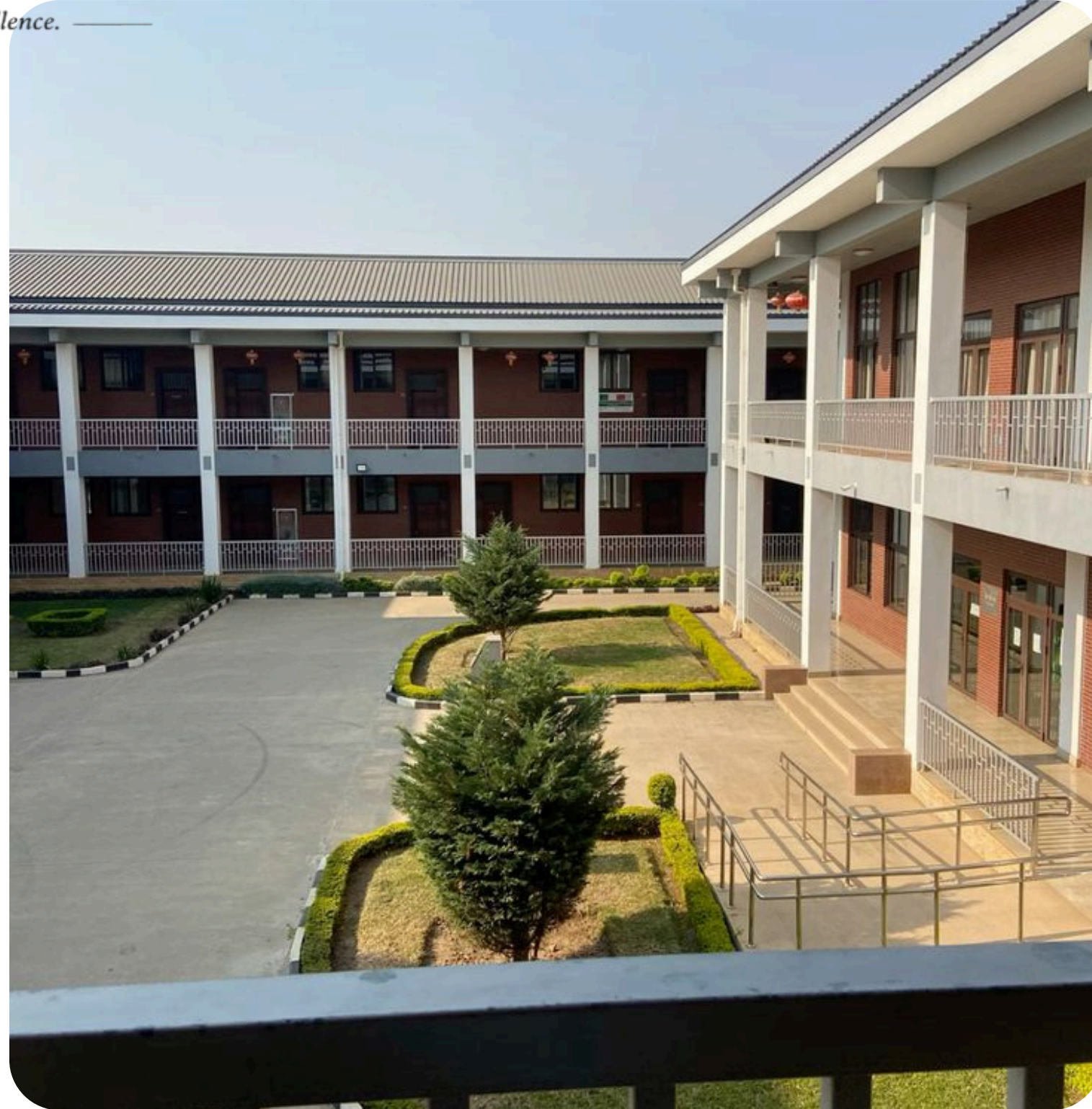
Project Type: School Building
