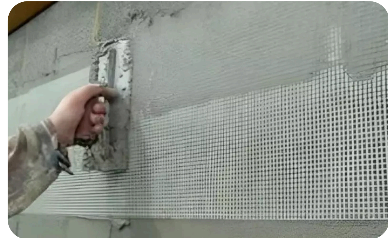
Plaster Mesh to protect walls
