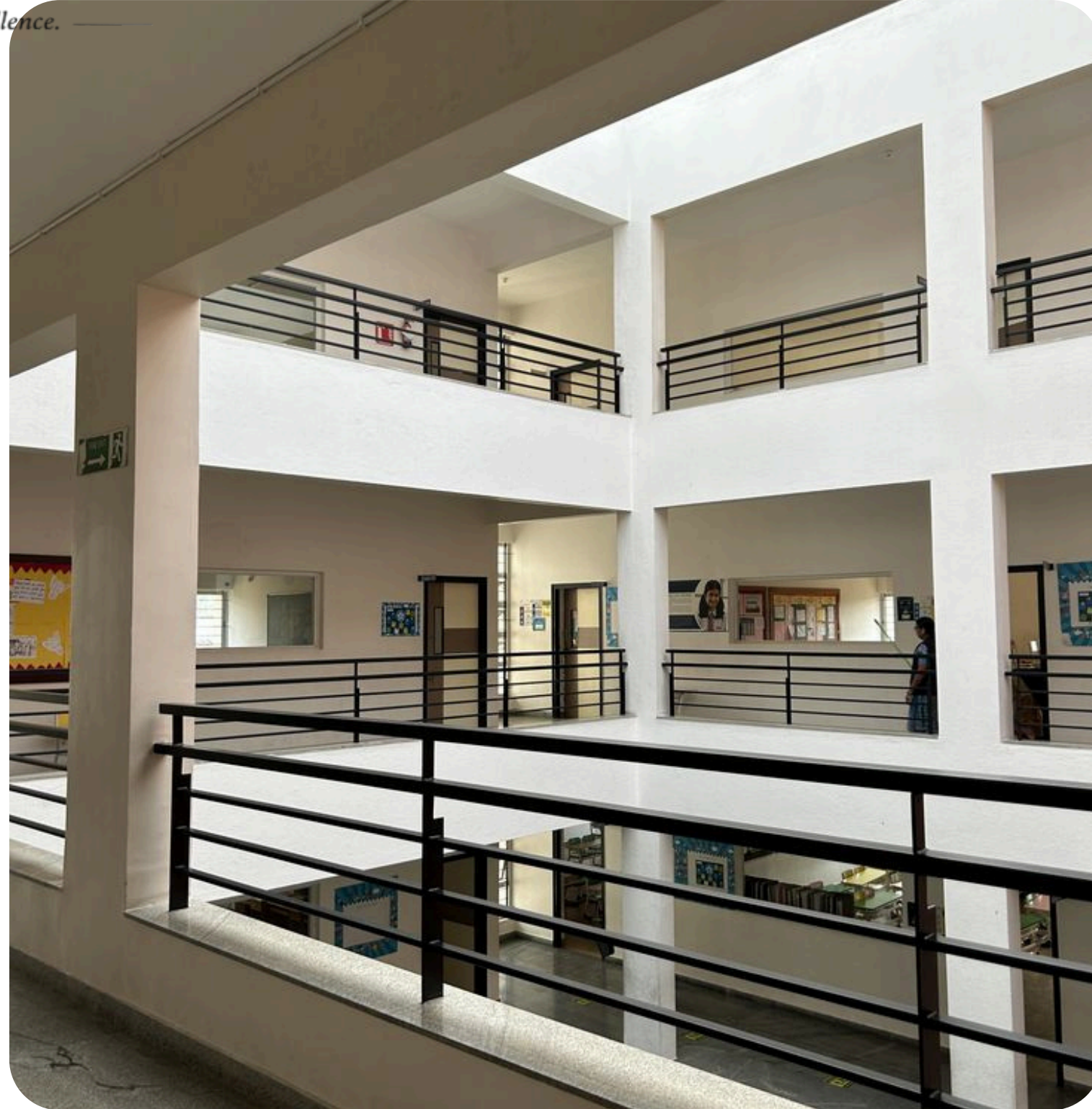
Project Type: School Building
