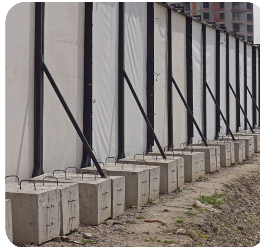
Temporary fencing and safety boundaries
