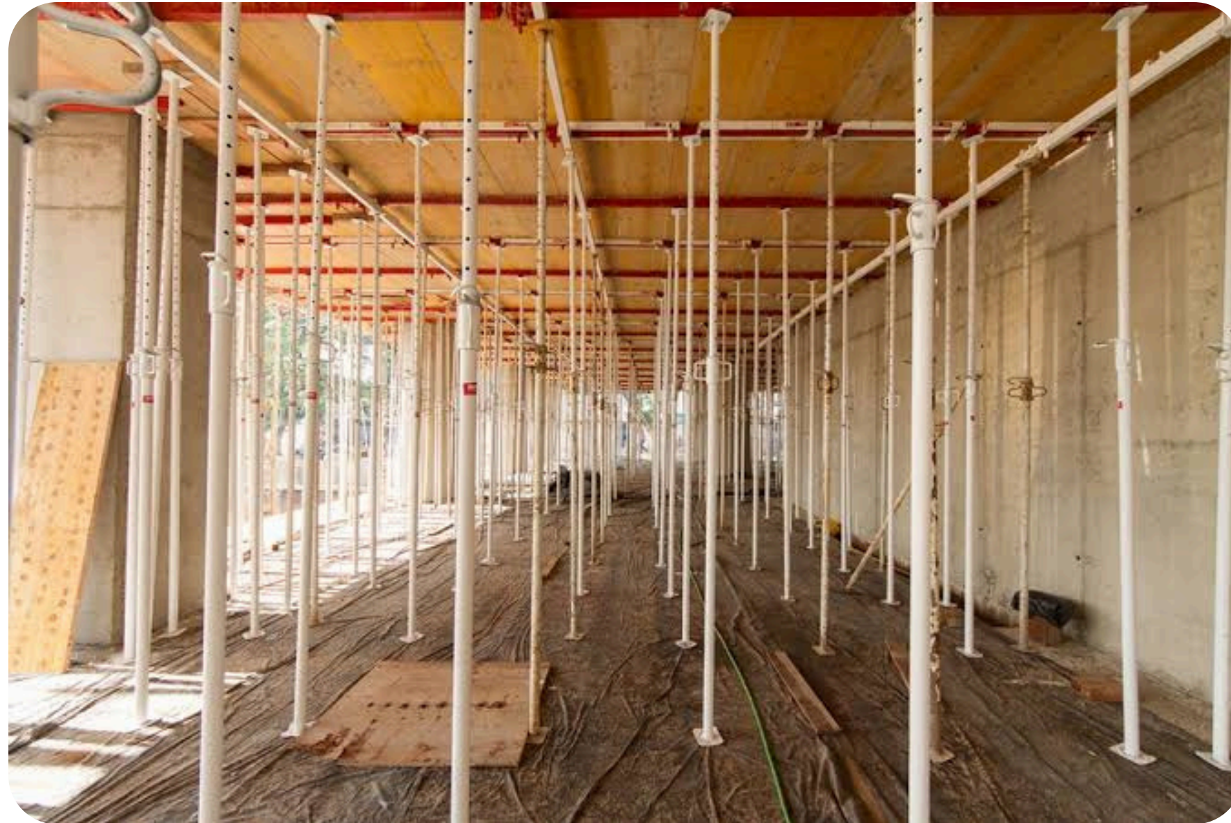
Formwork Installation for Slab
