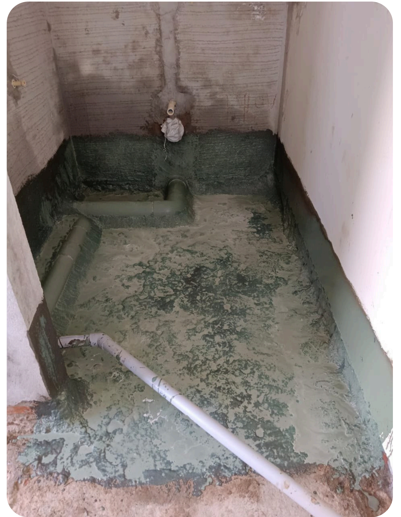
Bathroom Waterproofing
