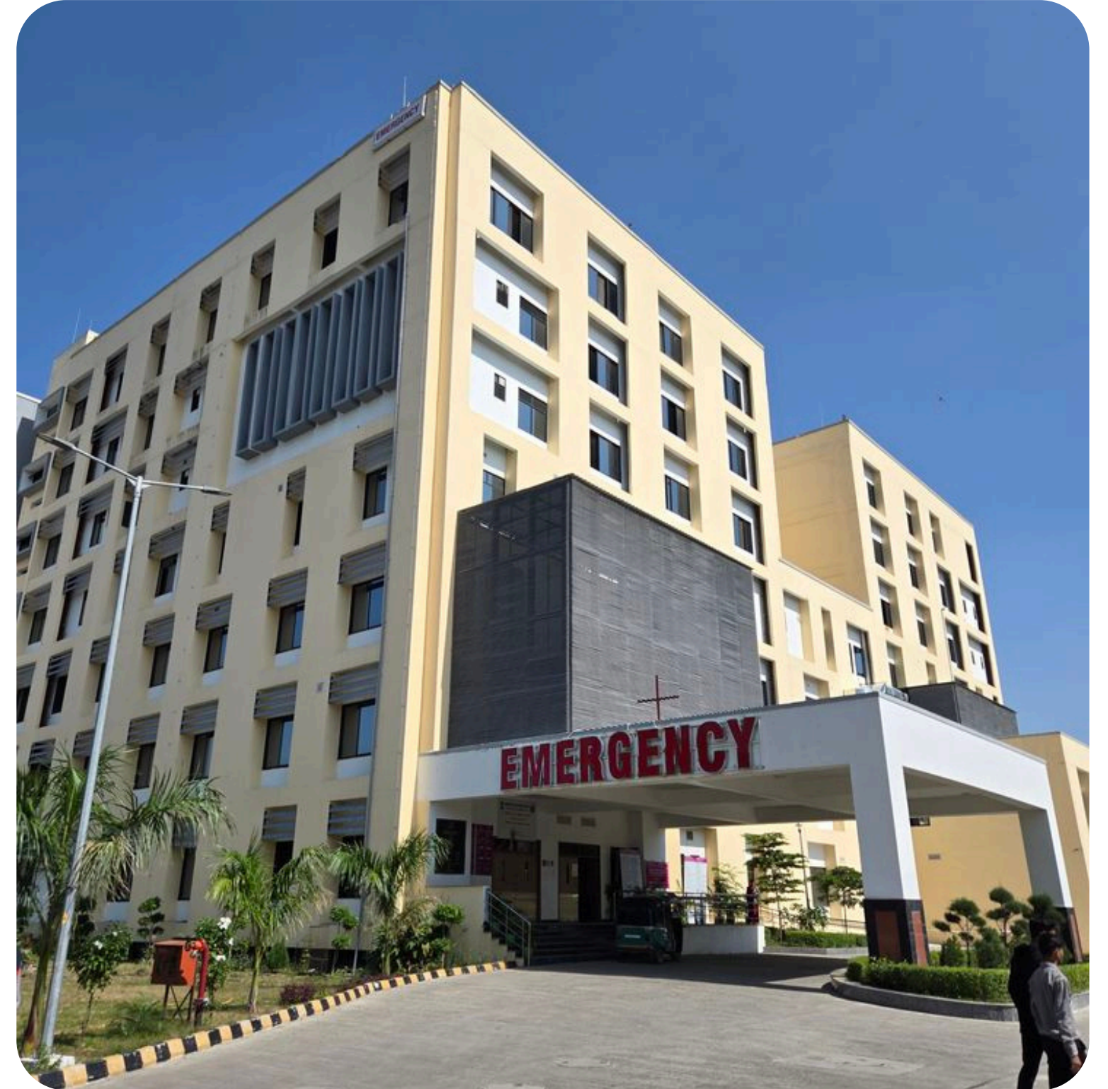
Project Type: Hospitals
