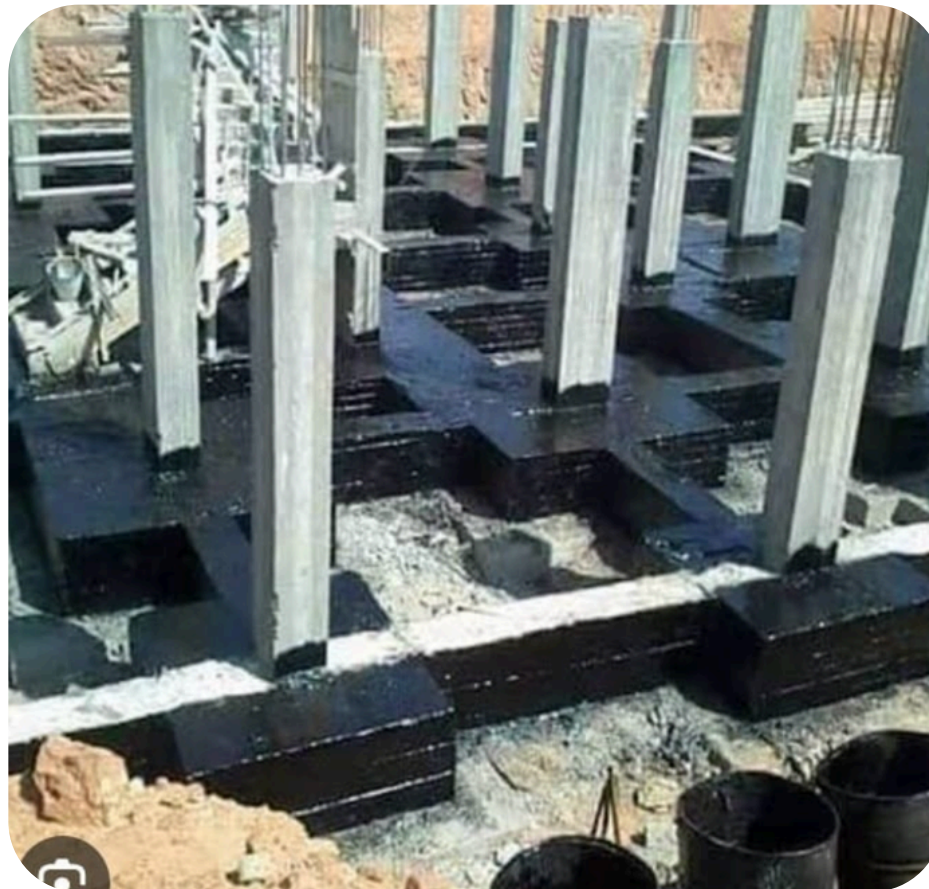
Bitumen Coating
