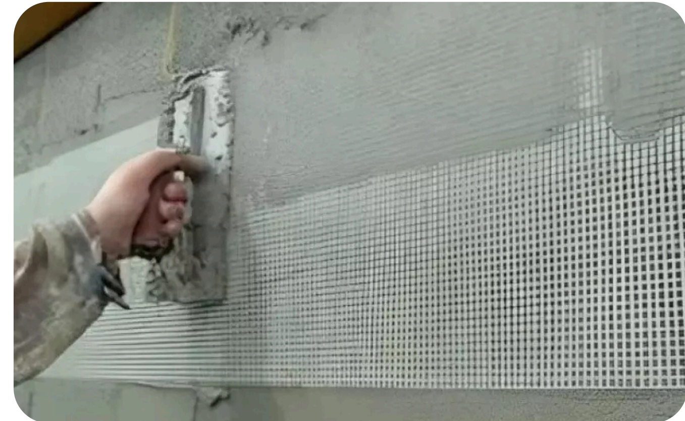
Plaster Mesh to protect walls
