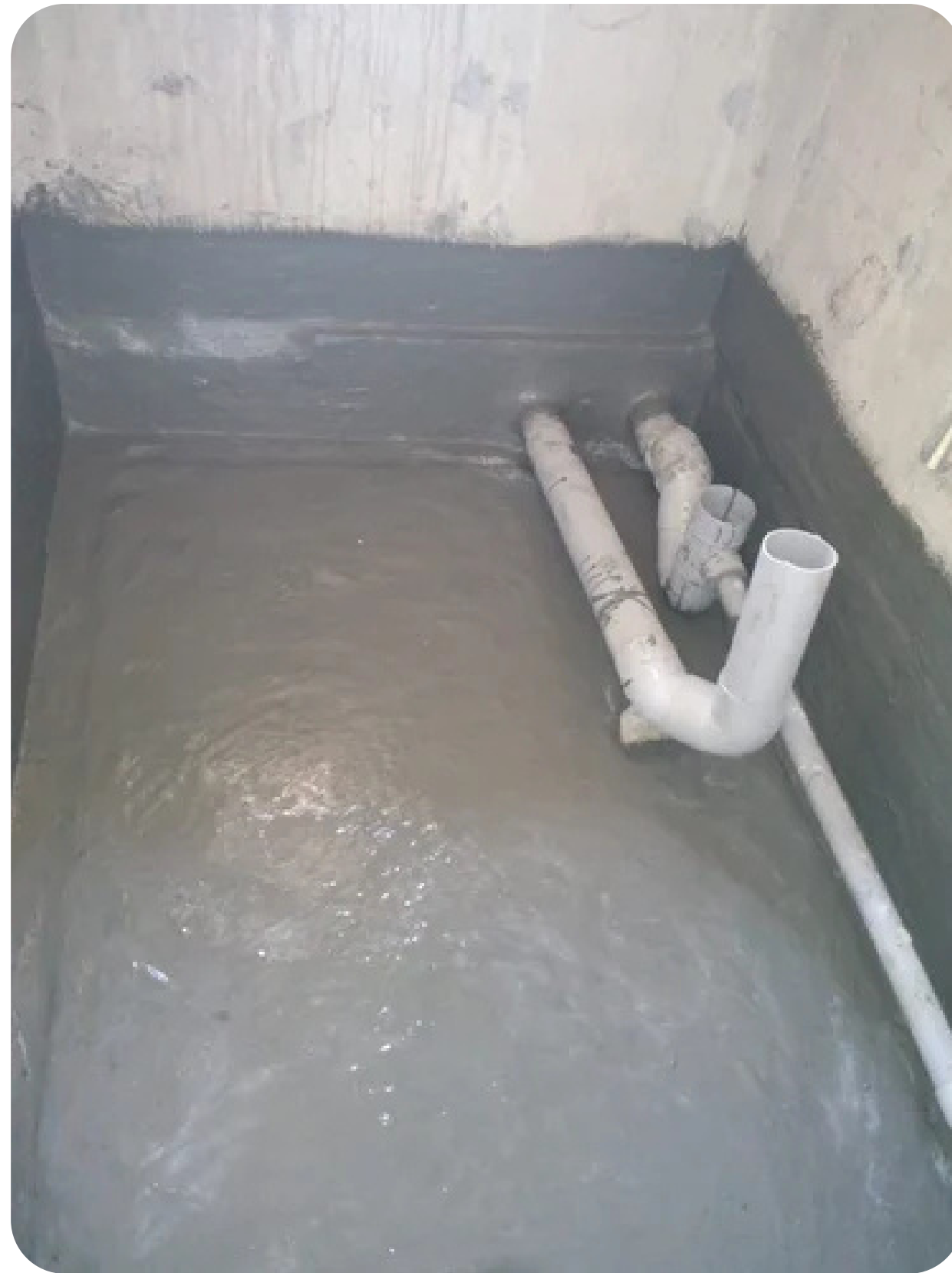
Bathroom Waterproofing
