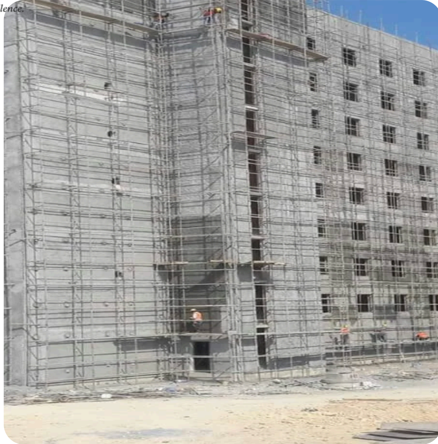
Project Type: Commercial Building
