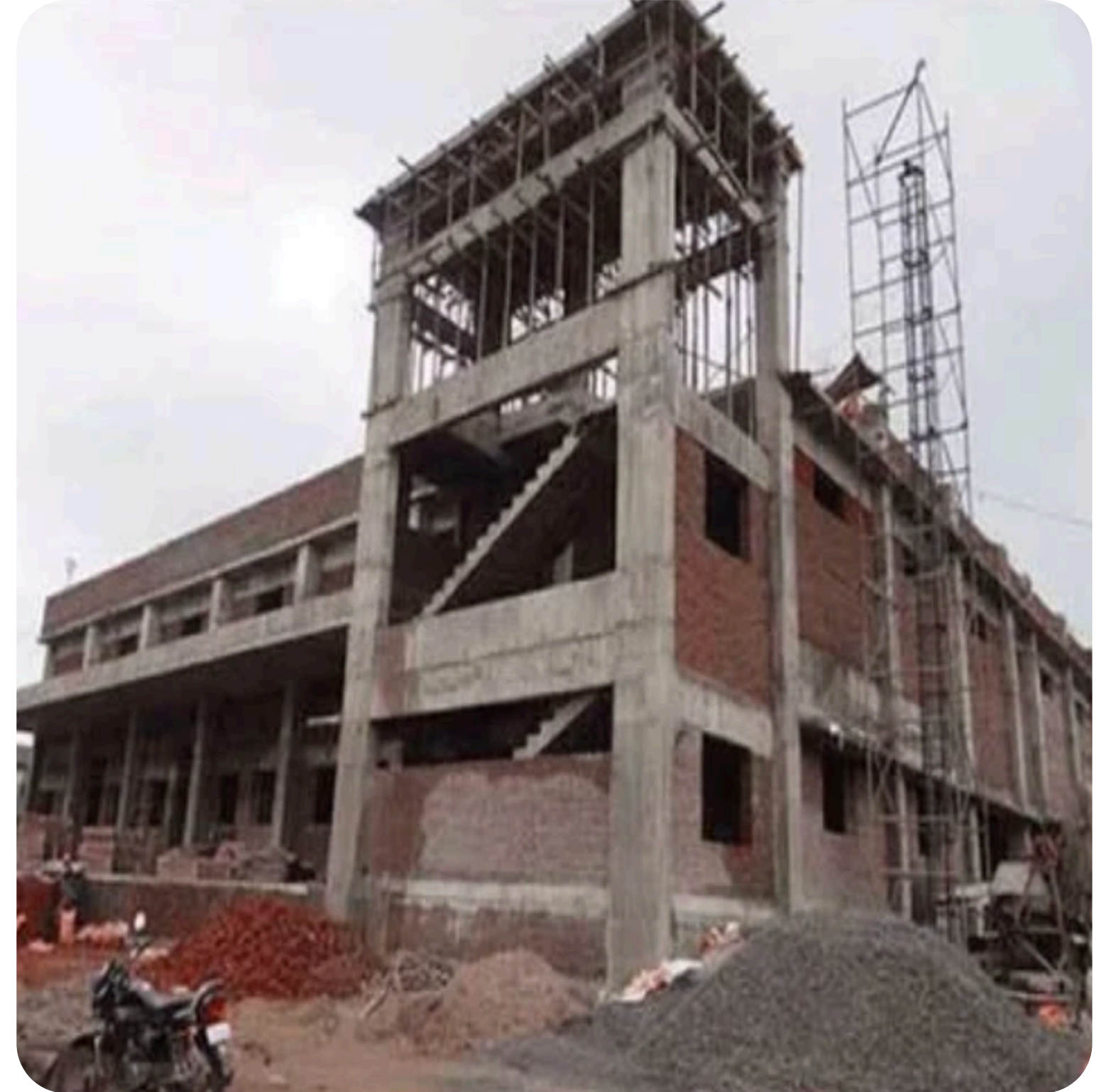
Project Type: Residential cum Commercial
